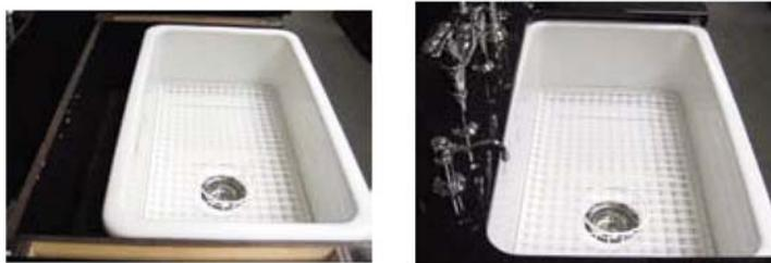
5. Design the cabinet frame separately from the cabinet fascia. The support frame or base should be designed to support the sink on the sides and the back. The cabinet trim that frames the sink can then be custom fit around the corners.
