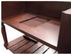
3. The most common installation design is undermounted below the solid surface. Using the sink to be installed, measure where to install the support frame. (Fig.1) Shimming may be necessary to move the sink up to the solid surface or to make the sink drain properly. A reveal of 1" to 2" inches is common. (Fig. 2)
