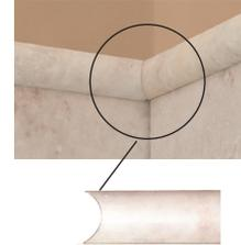
The solid surface bullnose molding used along the top edge of the walls is contoured for easy fitting.
