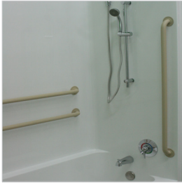
Grab bar and valve placement correctly placed and securely installed
