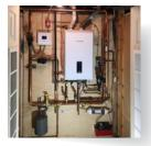
Compact NCB-E design fits well in tight spaces unlike a bulky, traditional boiler and tank hot water heater.
